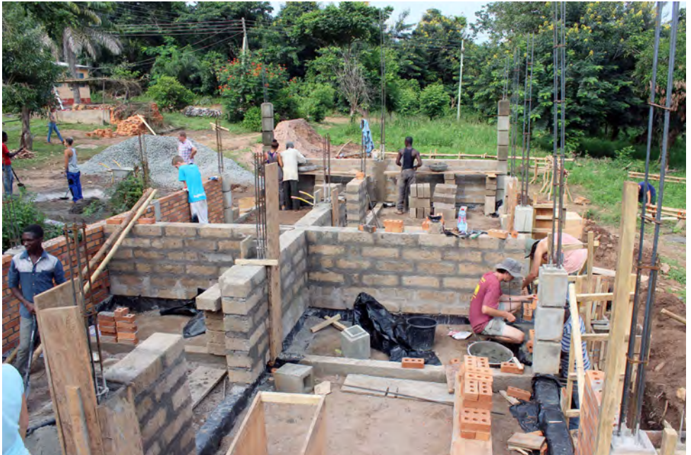
Baustelle / building site (mudbricks)
